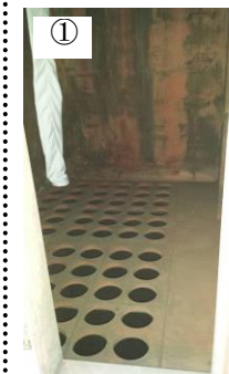
吊枠補修、室内清掃
